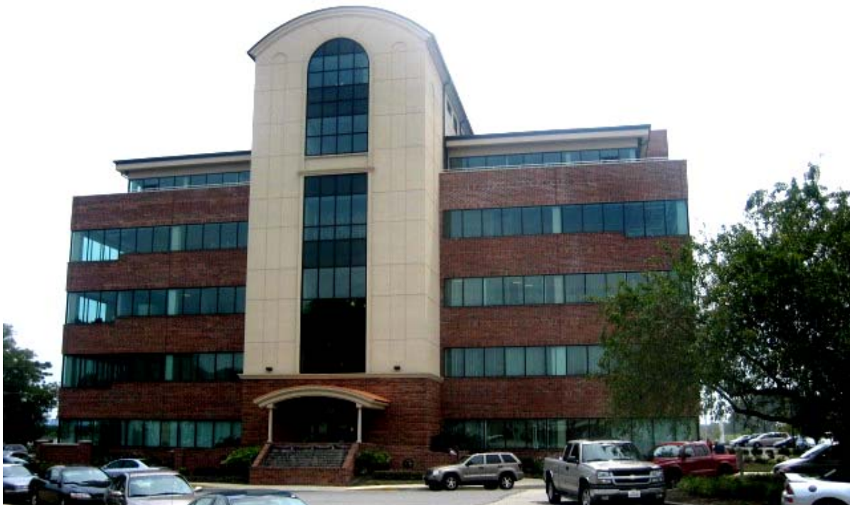
Figure 1: The Duncan Center, Personal Photo: Taken August 16, 2007
